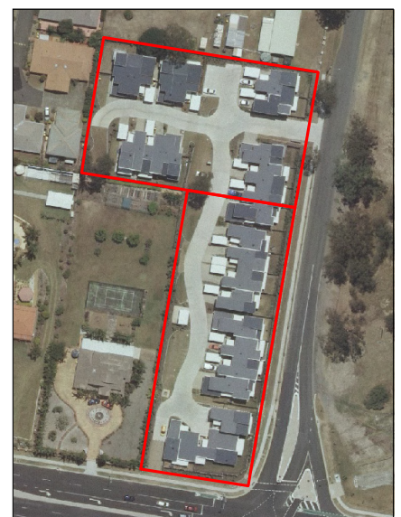
Figure 4 Aerial imagery flown mid to late 2009 showing completed development
